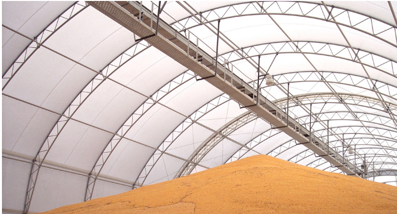
Horizontal drag conveyor in a flat storage application.
