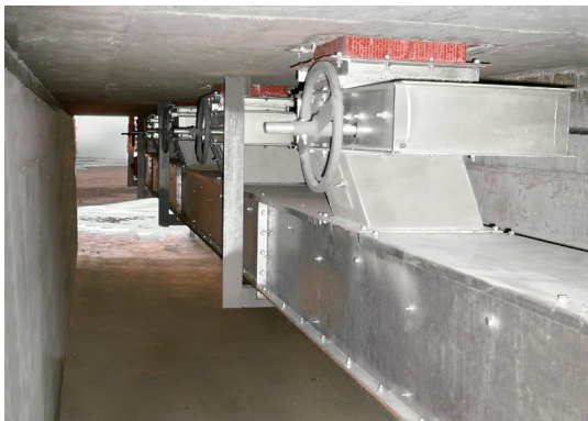
Drag conveyor installation in a trenched commercial bin floor.
